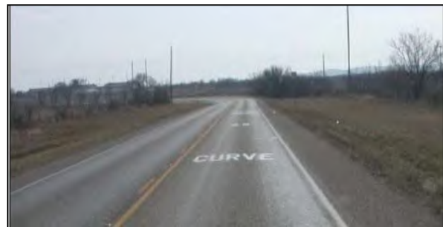
Figure 13. Photo. Pavement marking for advanced curve warning.
