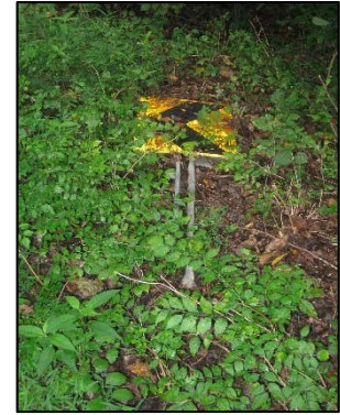
Figure 37. Photo. Example of a Chevron sign on the ground.
