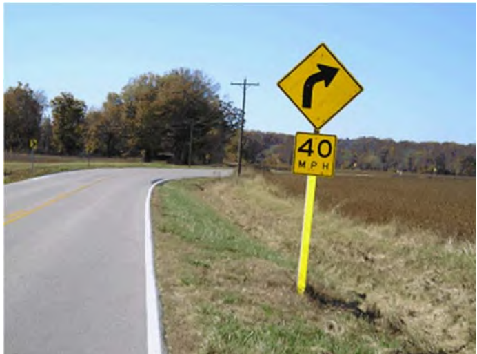
Figure C-1. Photo. Application of edge line at a horizontal curve.
