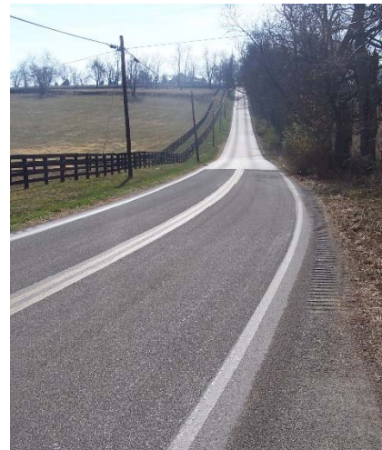
Figure F-2. Photo. A horizontal curve with HFST.
