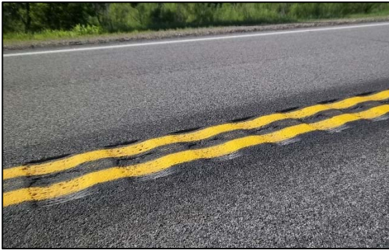
Figure 47. Photo. Milled Center Line Rumble Stripes.
