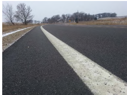
Figure 7. Photo. Delineation with enhanced (6-inch) edge lines.
