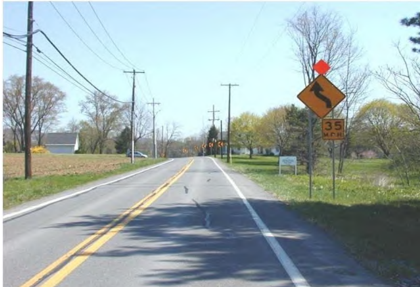
Figure A-1. Photo. An orange flag supplementing the reverse curve warning sign and speed advisory plaque. Chevrons were also used to delineate the curve.
