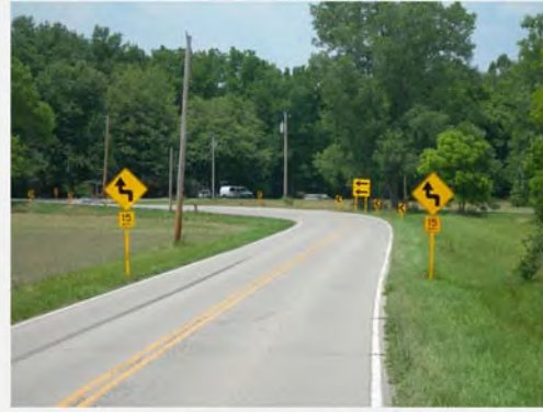
Figure 28. Photo. After signage updates.
