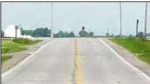
Figure 23. Photo. Before, without chevrons.
