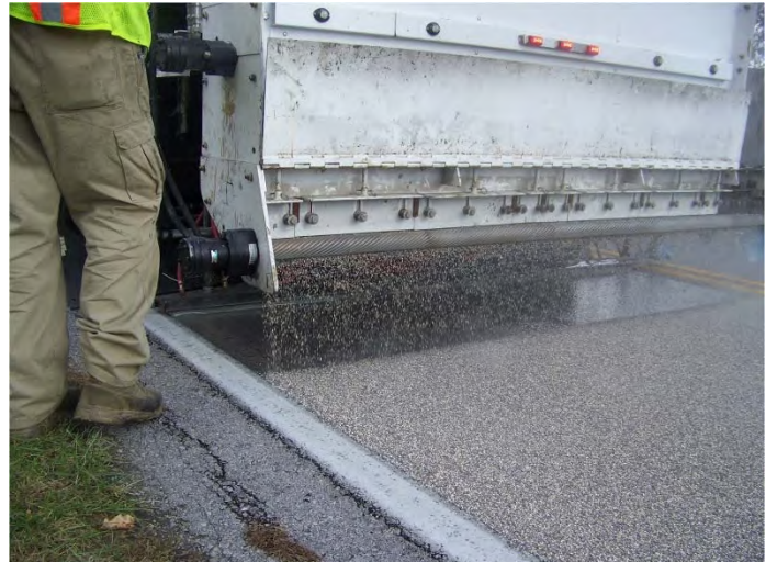
Figure F-1. Photo. A truck in the process of applying HFST to a curve.
