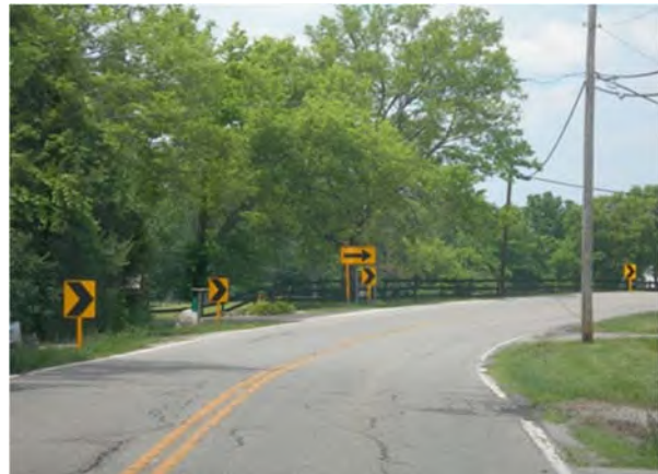
Figure D-4. Photo. A curve on a rural, two-lane road after signage updates through the Horizontal Curve Program.
